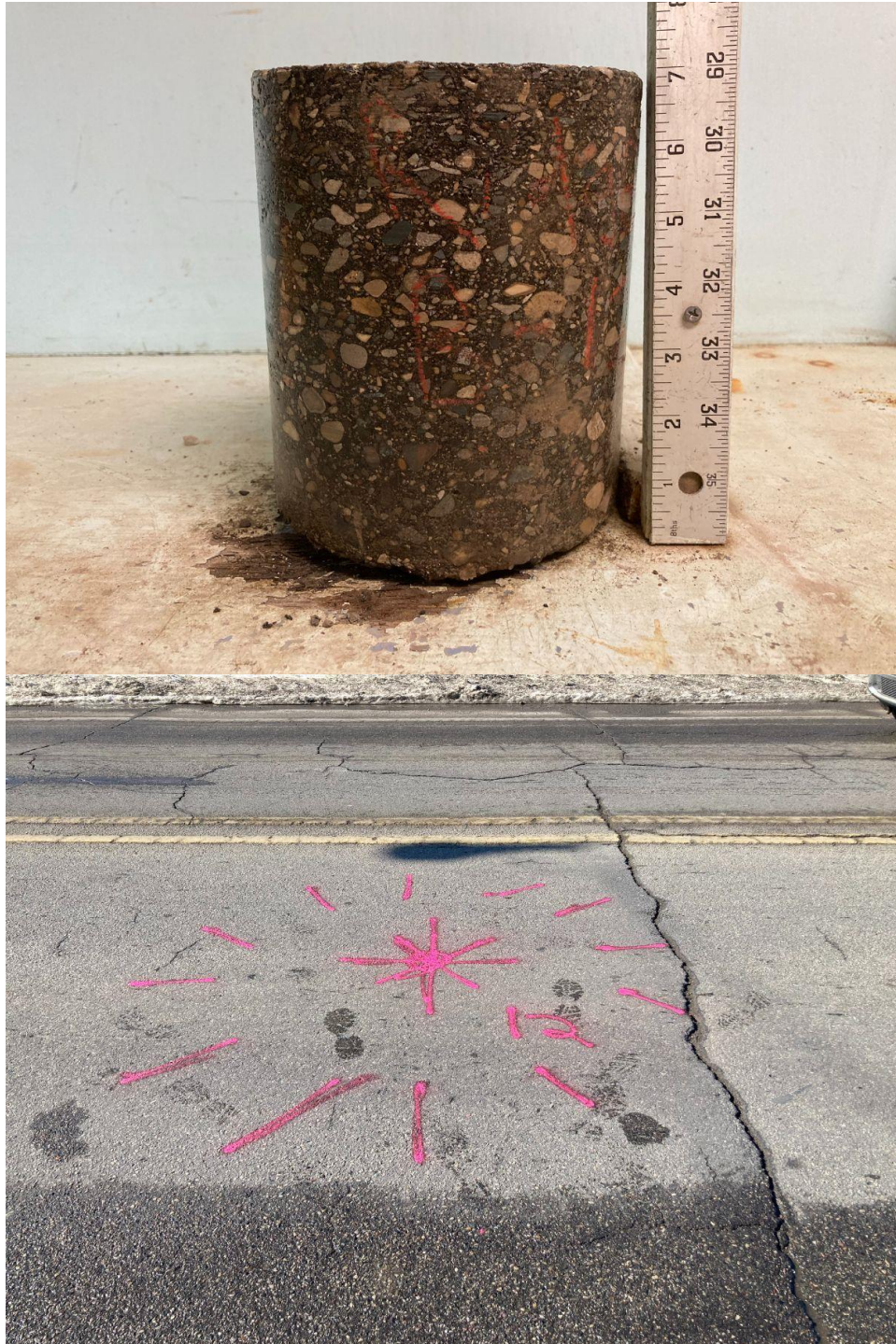
Core Photograph of B-12: HMA Pavement = 7 inches
