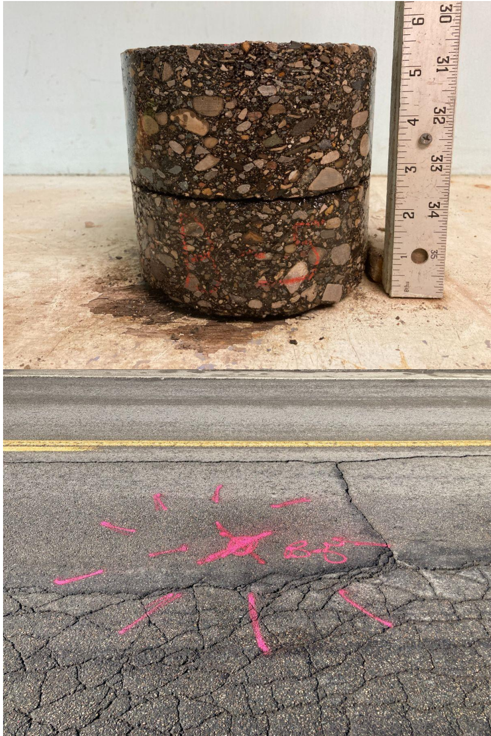
Core Photograph of B-05: HMA Pavement = 5-1/2 inches
