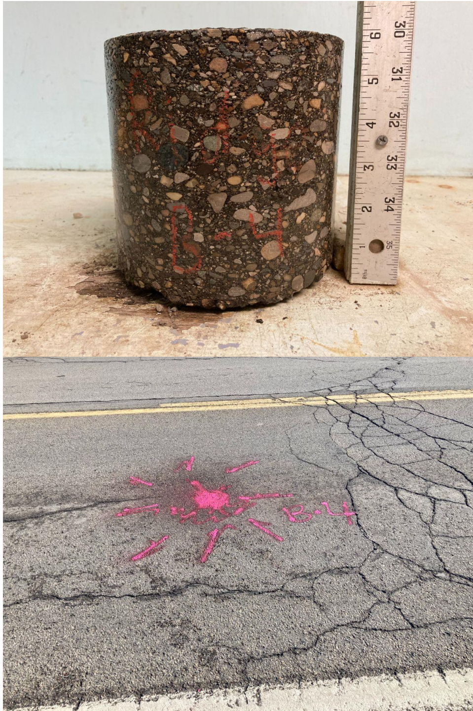
Core Photograph of B-04: HMA Pavement = 6 inches
