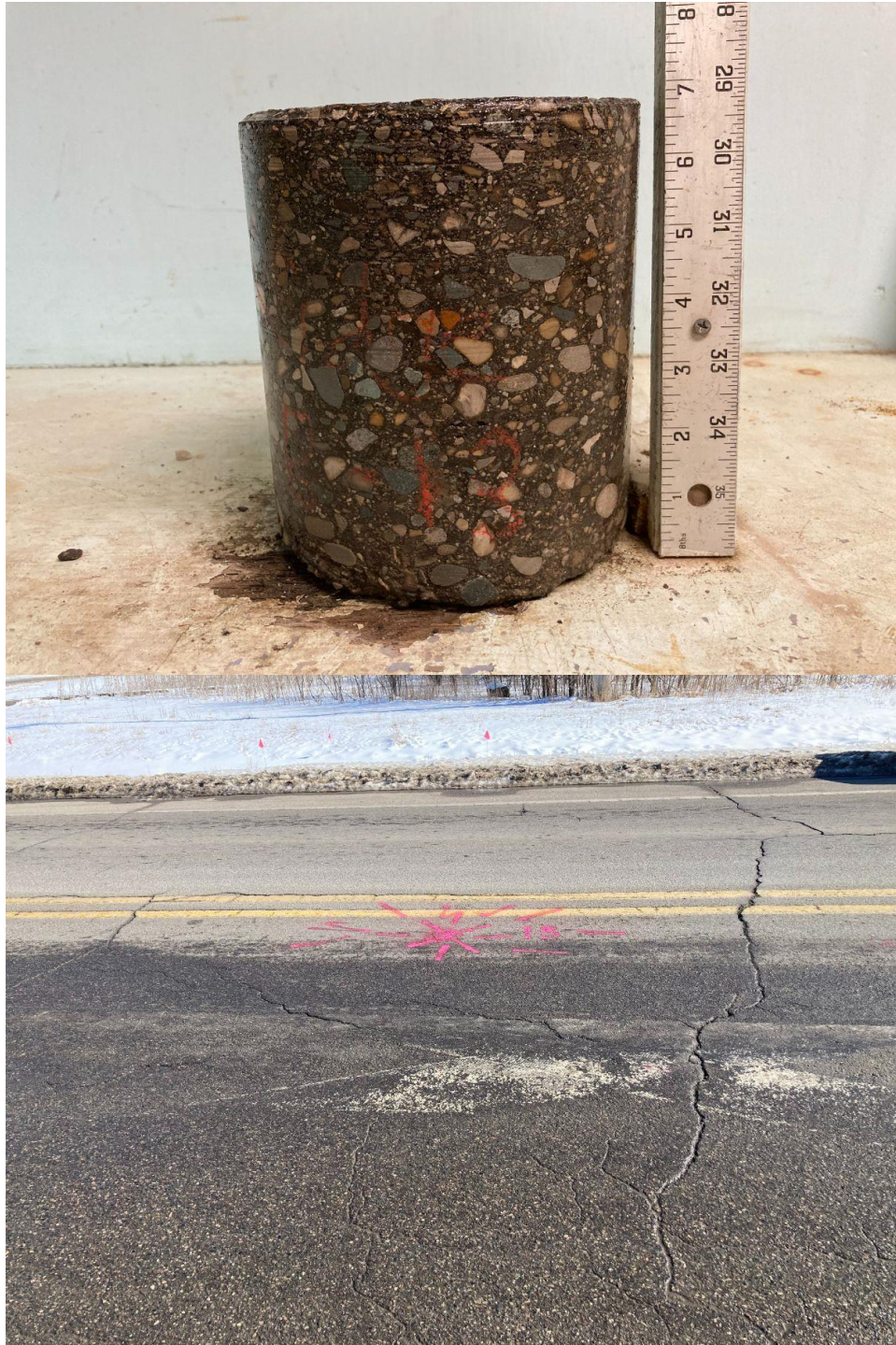
Core Photograph of B-13: HMA Pavement = 7 inches
