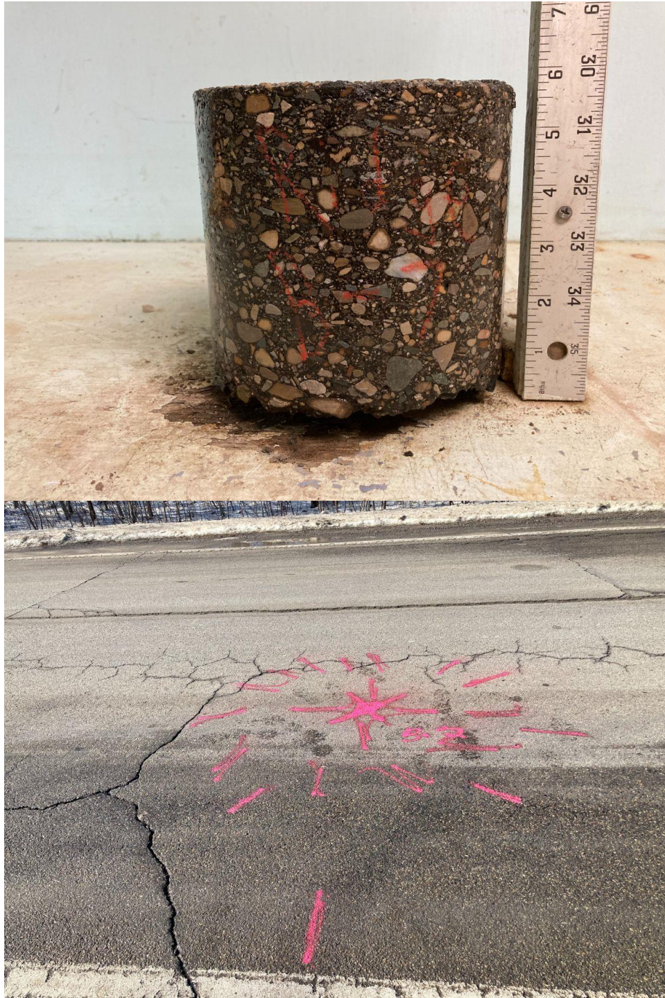
Core Photograph of B-07: HMA Pavement = 5-3/4 inches
