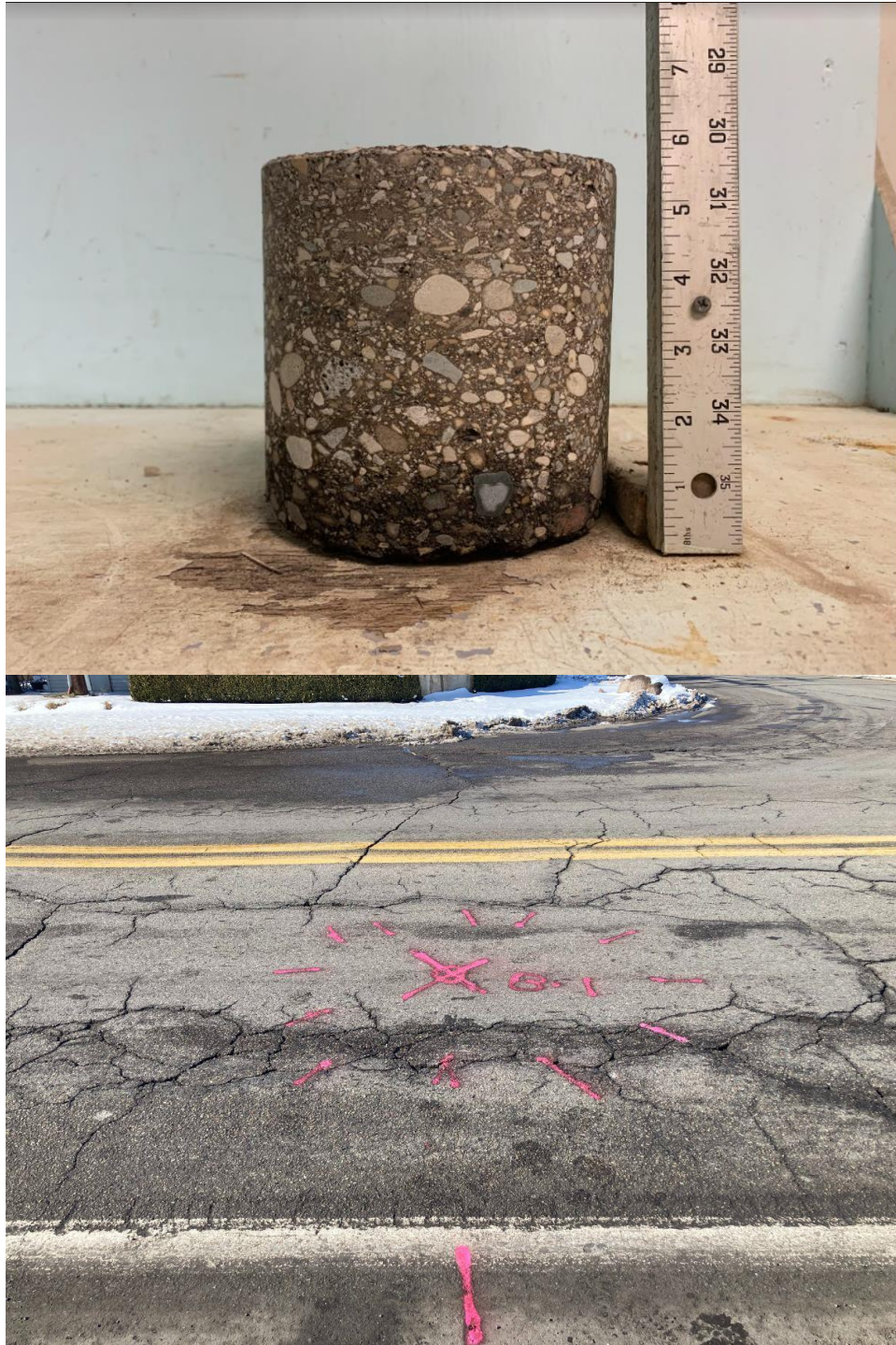
Core Photograph of B-01: HMA Pavement = 5-1/2 inches
