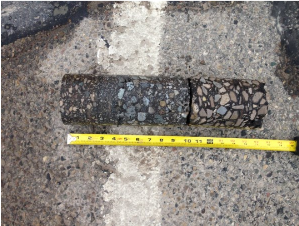
Core Photograph No. 5: 15 inches of Bituminous Concrete
