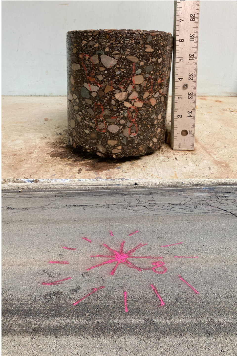
Core Photograph of B-08: HMA Pavement = 6-1/4 inches
