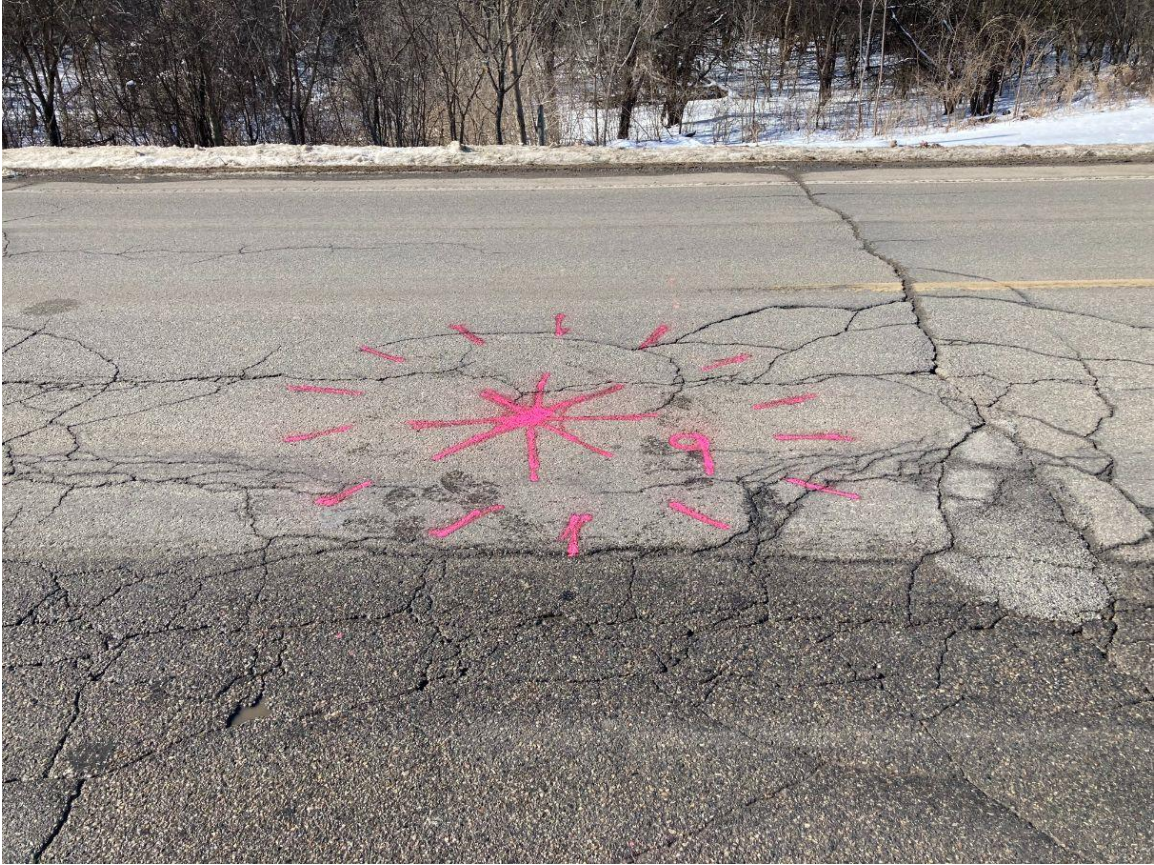
Core Photograph of B-09: HMA Pavement = 6 inches
