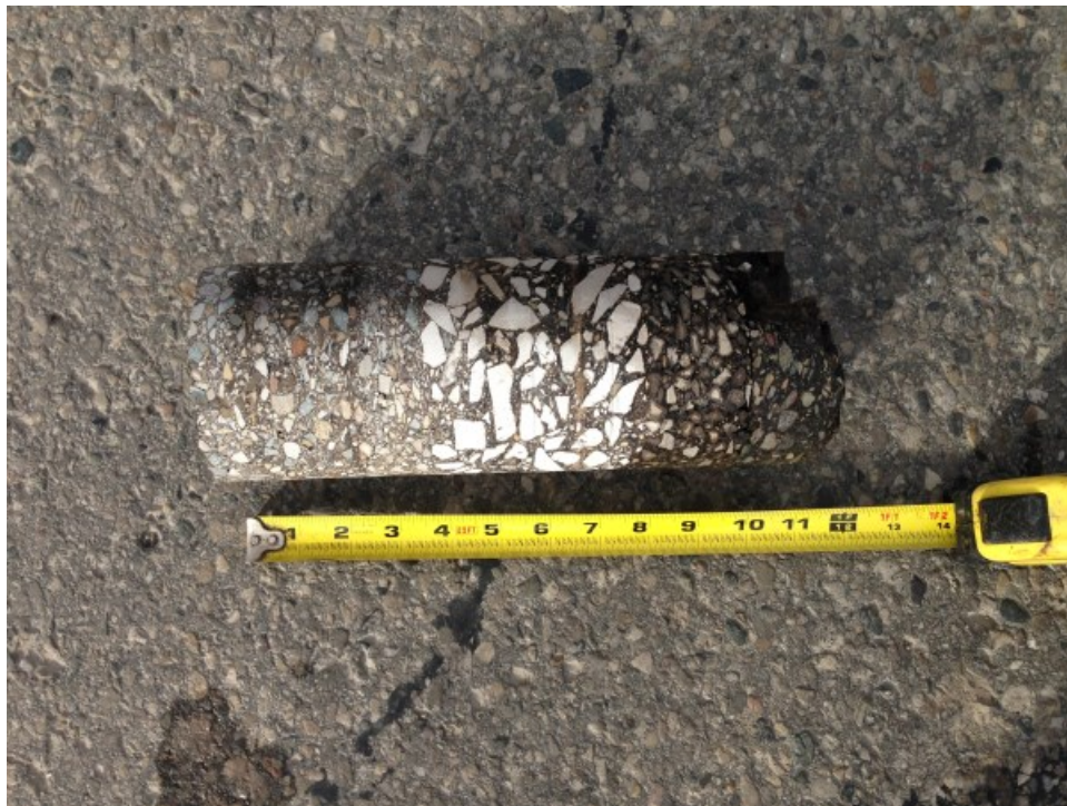
Core Photograph No. 4: 11 inches of Bituminous Concrete
