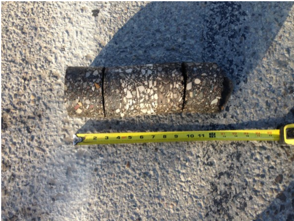
Core Photograph No. 2: 12 inches of Bituminous Concrete
