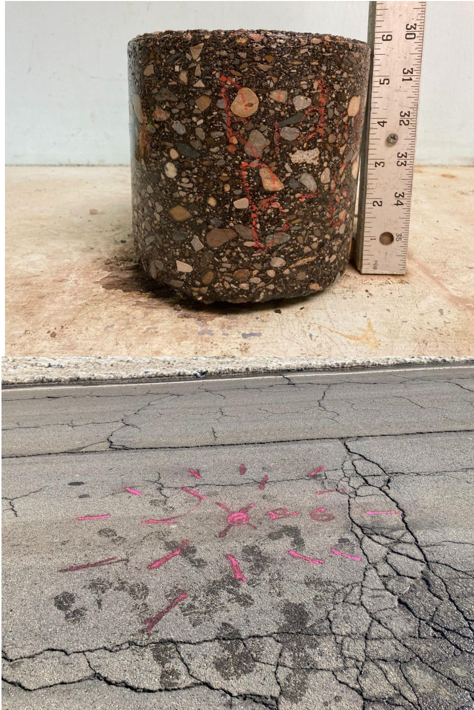
Core Photograph of B-06: HMA Pavement = 5-3/4 inches
