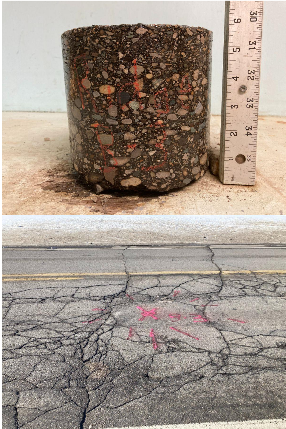
Core Photograph of B-03: HMA Pavement = 5-1/2 inches
