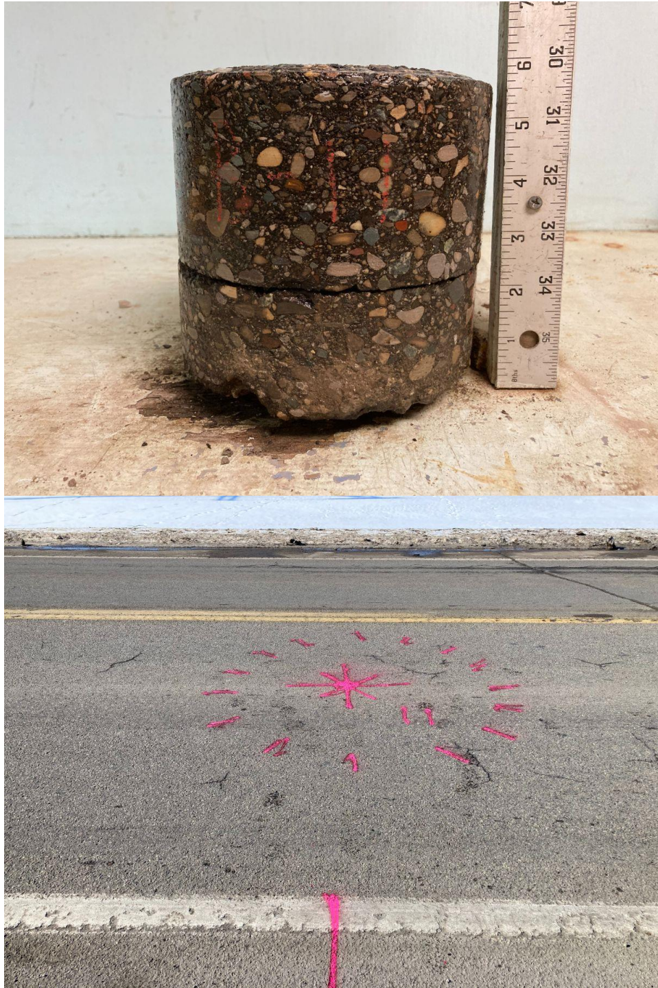
Core Photograph of B-11: HMA Pavement = 6 inches
