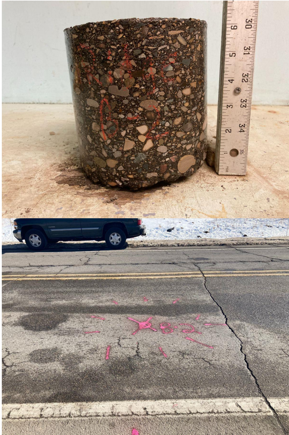
Core Photograph of B-02: HMA Pavement = 6 inches
