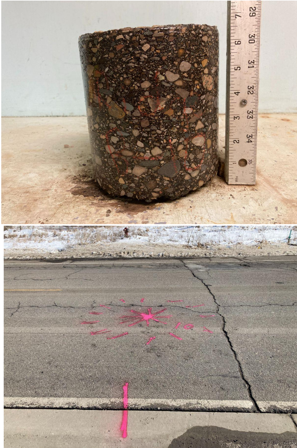
Core Photograph of B-10: HMA Pavement = 6-3/4 inches
