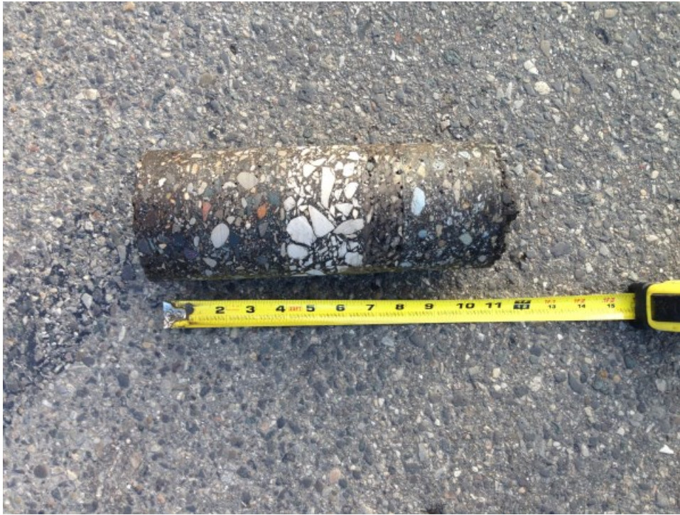
Core Photograph No. 1: 10-1/2 inches of Bituminous Concrete
