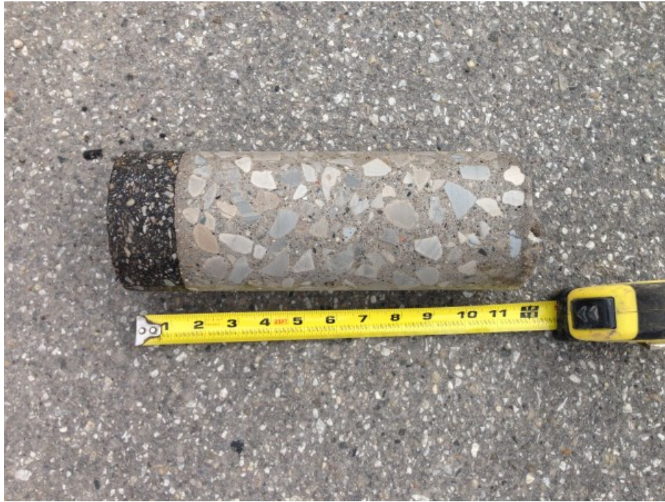
Core Photograph No. 9: 1-3/4 inches of Bituminous Concrete 9-1/4 inches of Portland Cement Concrete
