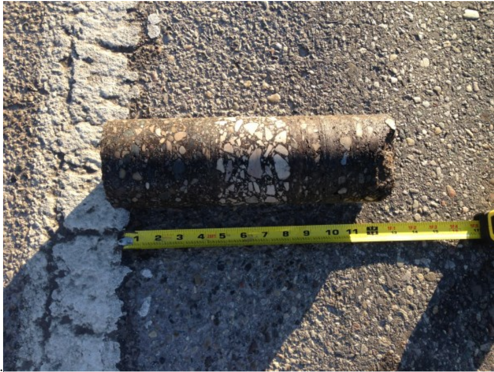
Core Photograph No. 3: 12 inches of Bituminous Concrete
